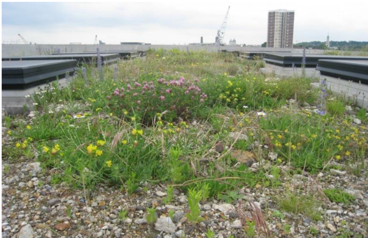
Figure 0-6: Example of naturally colonising brown roof on similar substrates to the Project Site
