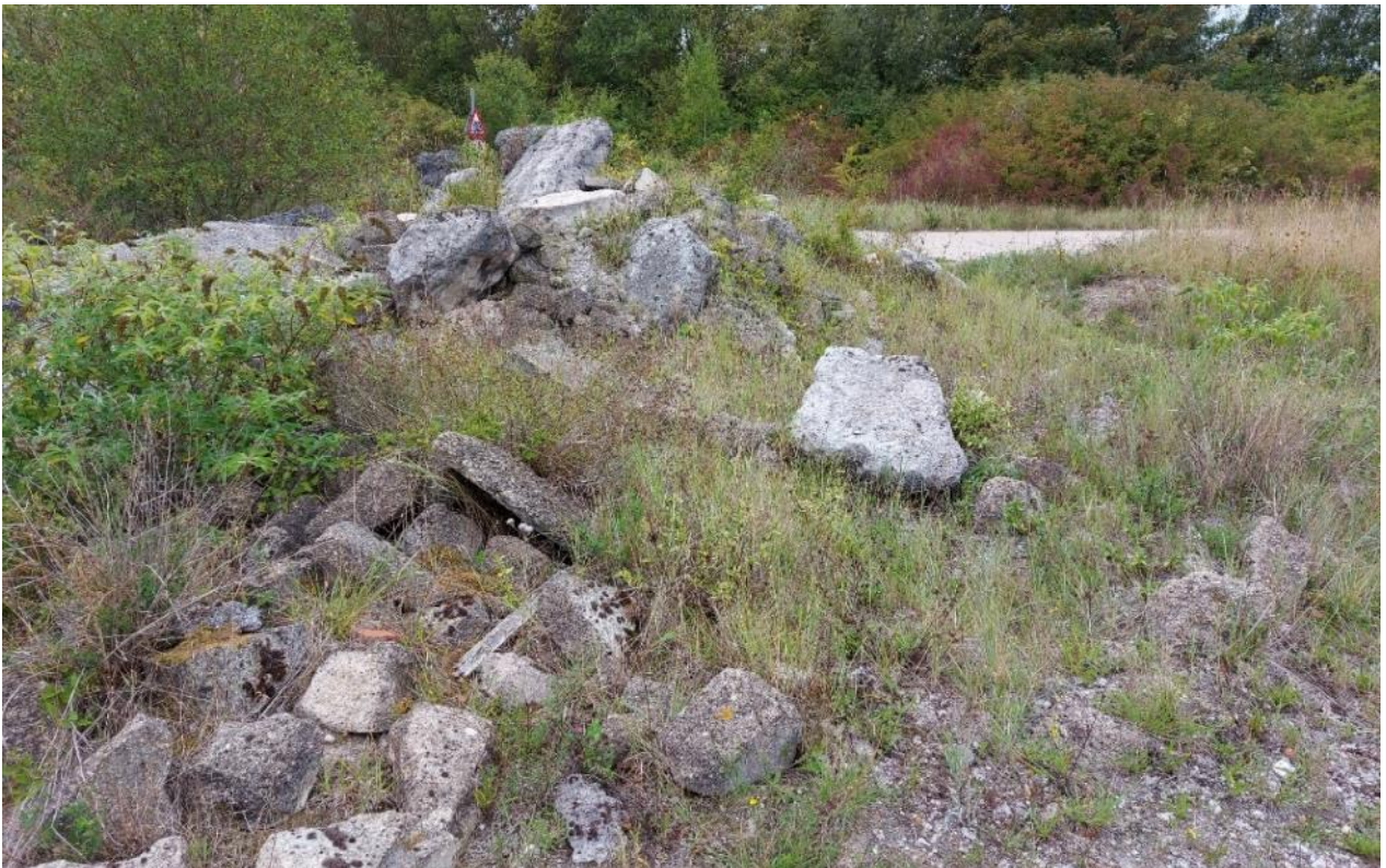
Figure 0-3: Example of existing mixed concrete rubble pile
