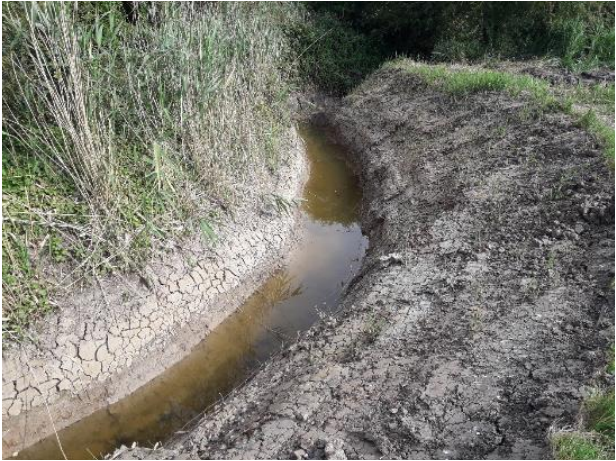
Figure A2-14: Dredging management in ditch D30. Stretches dredged on rotation
